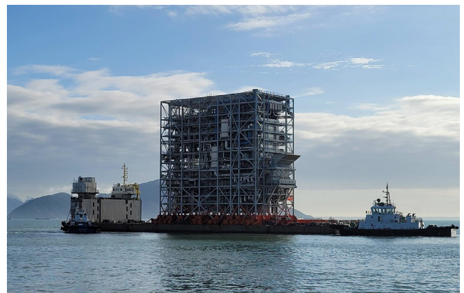
Shipment of 6,000 tonnes / 18 storey high construction module
