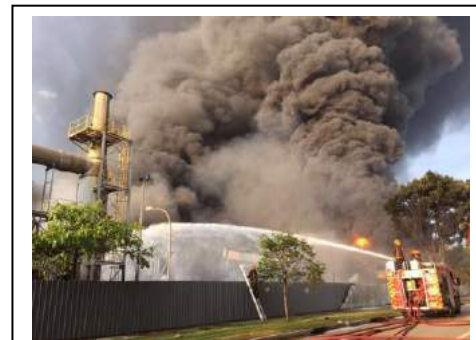
A damaging fire at a waste management plant
